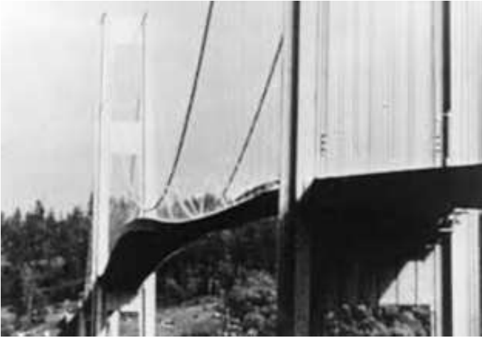
Figure 5.5 – The Tacoma Narrows Bridge
