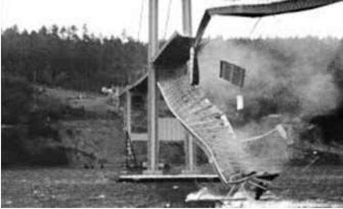
Figure 1.4 – The Tacoma Narrows Bridge collapse
