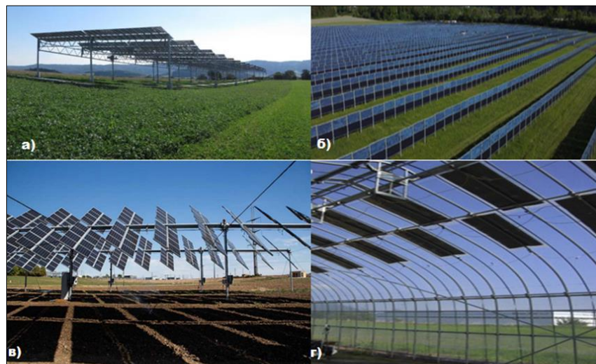
Figure 2.4 – Possible types of placement of photovoltaic panels a) straight rows, b) in a checkerboard pattern, c) at an angle, d) vertical [22, 23, 24]
