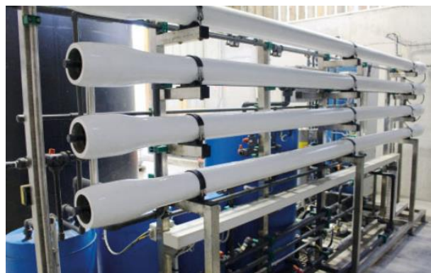
Figure 7 – Membrane filtration process with reverse osmosis modules [3]
