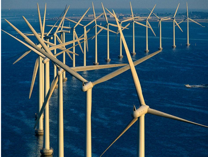
Fig.1 – Example of installations.
