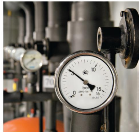
Figure 12.9 - (a) A Bourdon pressure gauge. When the pressure inside the flexible tube increases, the tube straightens out a little, deflecting the attached pointer. (b) This Bourdon-type pressure gauge is connected to a high-pressure gas line. The gauge pressure shown is just over 5 bars (1 bar = 10 5 Pa)
