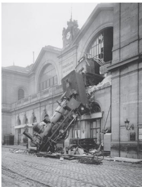
Figure 1.2 - This spectacular mishap was the result of a very small percent error - traveling a few meters too far at the end of a journey of hundreds of thousands of meters
